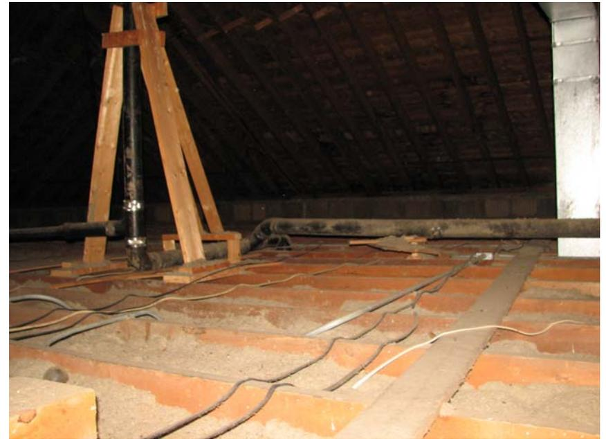
Attics are a great place to see construction materials used the building but which may be covered. The ceramic tiles above can also be seen in a wall cavity in the basement and behind the stairs in the large stairwell.
