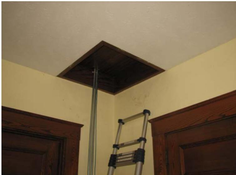
For attic work, this hatch will need to be converted to a folding attic stairwell, covered by a gasketed thermadome. I think installing near the back of the balcony section might be best and then sealing this access of completely.
