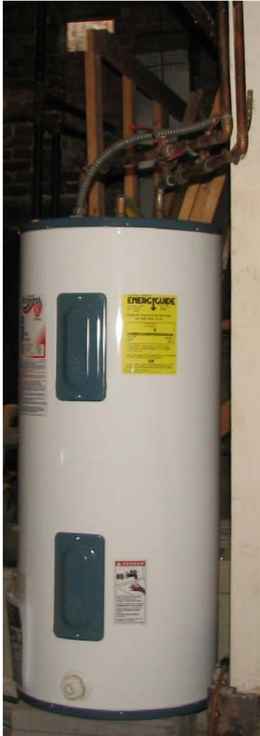
Presumed that hot water use is minimal....switching to a tank less water heater will definitely reduce energy use, especially in the summer. But hard to project savings since this tank isn't metered. In general – heating water to be stored hot – especially when not called upon very often - is not an efficient use of energy.
