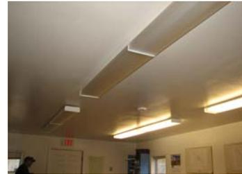
Ceiling has 6”batts on strapping with poly layer underneath – so fiberglass is not in direct contact with any air barrier. Effective R10-15 at best. Very small, vented attic space. Low pitch roof with 2x4 truss won’t allow for snow loads, so roof has to be shoveled.
